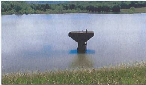
Principal Spillway Intake Tower
