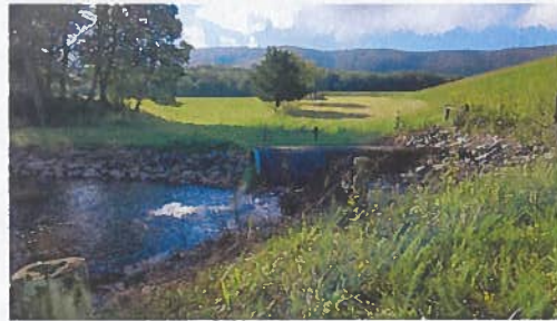
Principal Spillway Outlet
